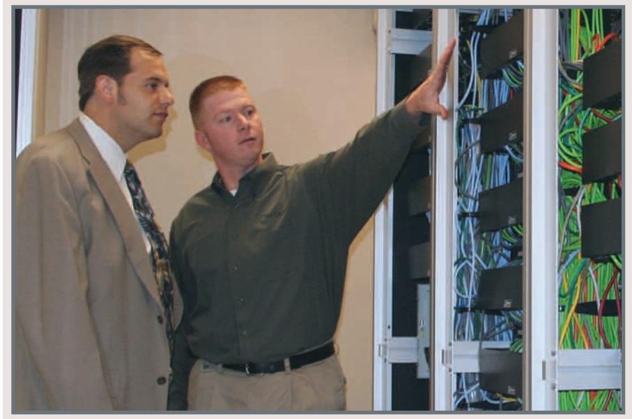
Lance Lelm, Vice President of Heart Technologies, shows Matt Hallam the extensive hardware housed in a separate room at Heart's headquarters in East Peoria.
